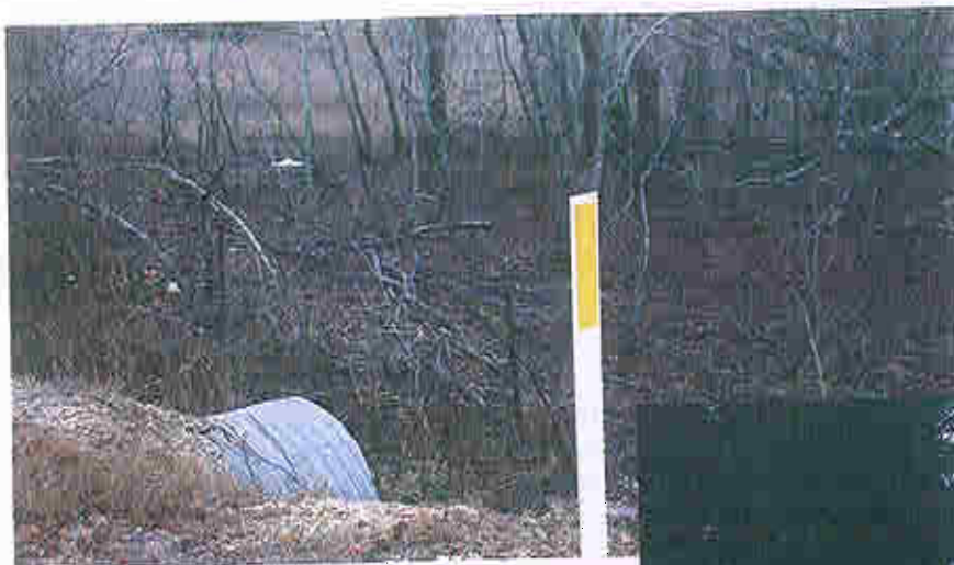
Type 2 object marker used to mark culvert end.
