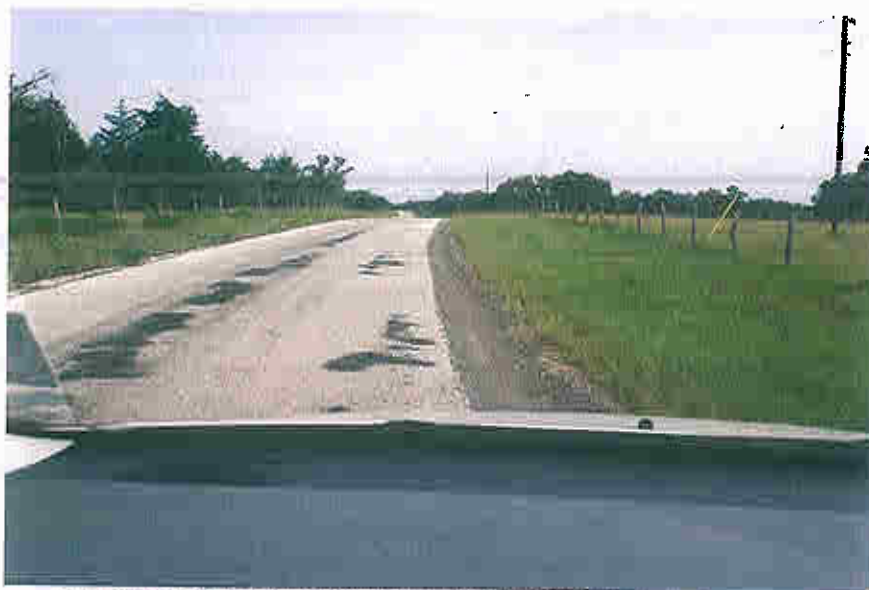
Keeping shoulders pulled up to the pavement edge avoids hazardous pavement edge drop-offs. Photos by Howard McCann, TEEX
