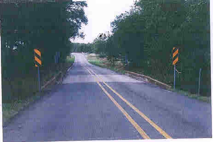
Type 3 object markers used to mark bridge ends.
